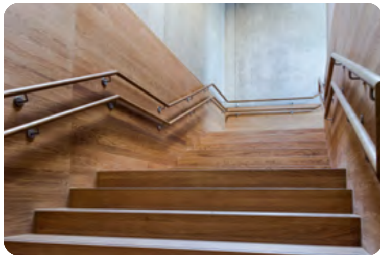
The combination of wood and exposed concrete as primary materials also characterizes the impressive stairway.
